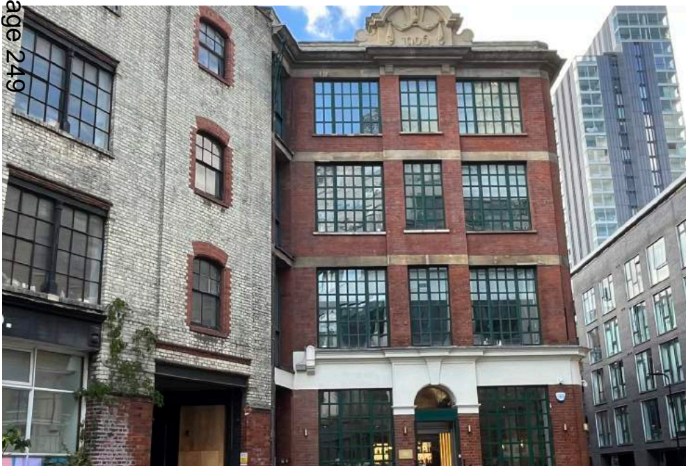
Top: View north on Westland Place Bottom: Pickwick House, Westland Place
