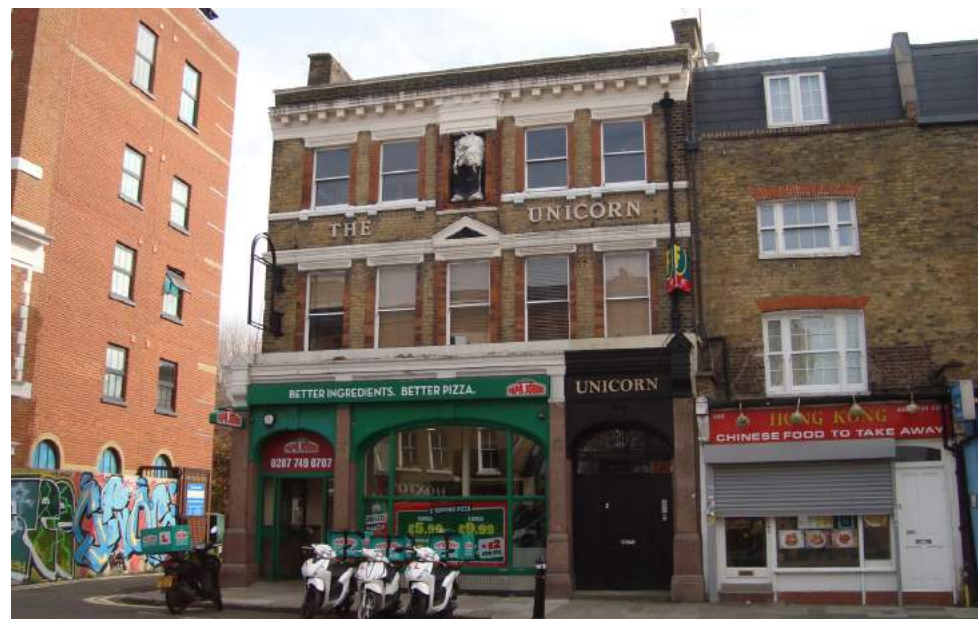
The former Unicorn pub at 202 Hoxton Street
