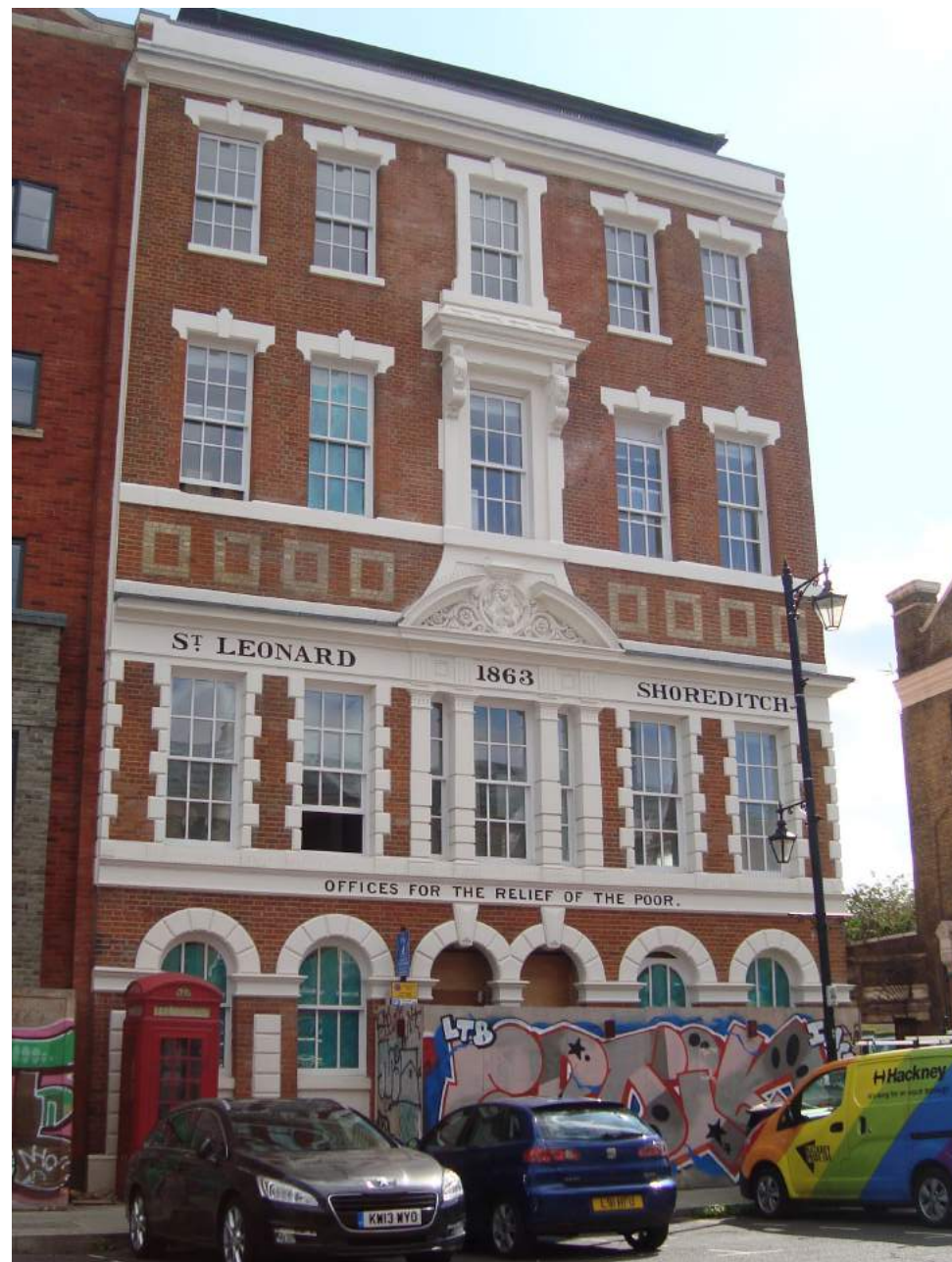
The facade of St Leonard Parish Relief Offices has been refurbished as part of a regeneration project for the wider hospital site
